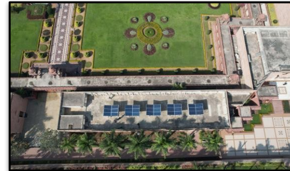
Akshardham Project India's First Portable Rooftop Solar Systems Installed at Akshardham Gandhi Nagar
