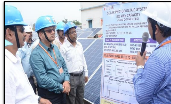
Rooftop Solar Project IOCL (Haldia & Panipat Refinery)
